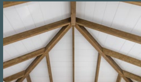
*exposed beam ceiling
