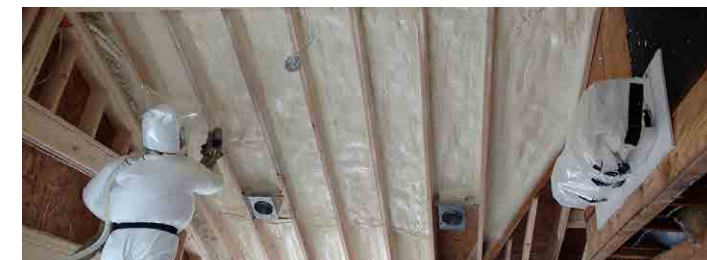
Spray Foam Insulated Floor
